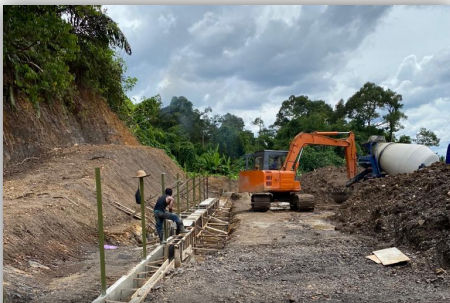
Factory Drainage Installation
